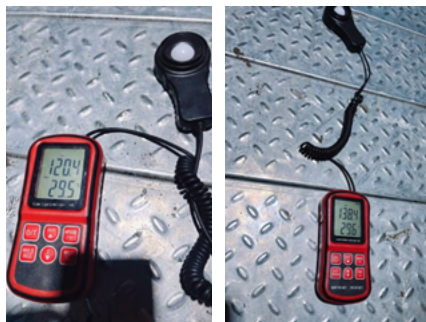
Ground Illuminance Before (Left) and After (Right) Lighting System Retrofit
